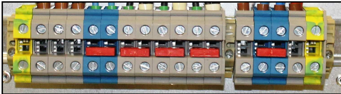
Figure 2.2 10-15-20-30 kVA Cable Connection
